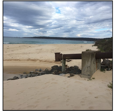
Waste water outlet as it is on Merimbula Beach today.
